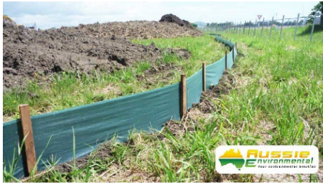
Geofabric fence, 300mm depth in trench, includes timber pickets at 3000mm centres
