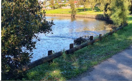
Timber post fence (half logs)
